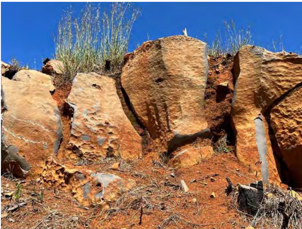
Photo 2: Closeup of blocks of the Paradise olivine basalt with residual soil between blocks. This is the PR soil unit of Wert & Associates (1992).
