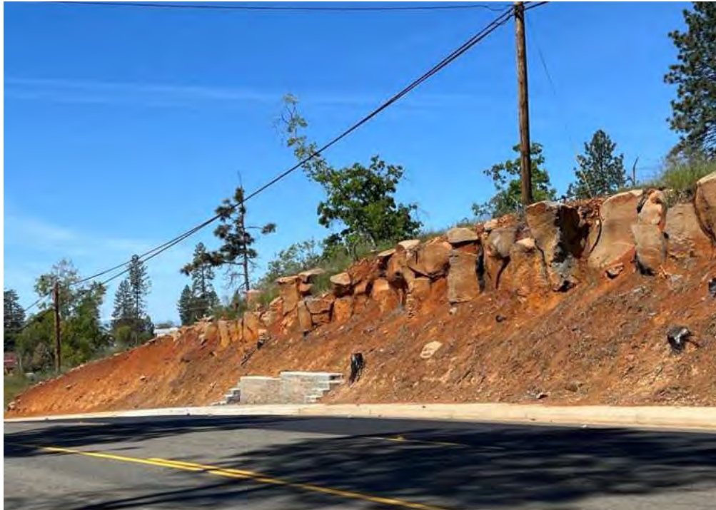
Photo 1: Road cut along Pearson Road exposes the Paradise olivine basalt over deeply weathered volcanic mudflows (lahars) (Tpb).
