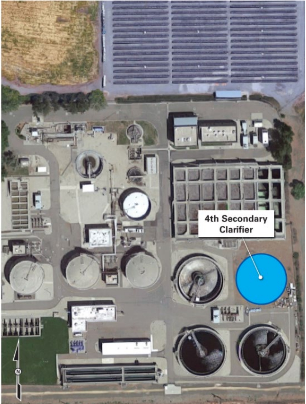
Figure 4.2 Fourth Secondary Clarifier
