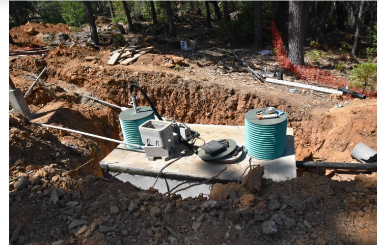
Septic Tank & STEP pipe
