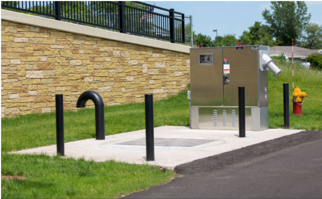
Figure 2-9. Example Transition Chamber with Vehicular Bollard Protection
