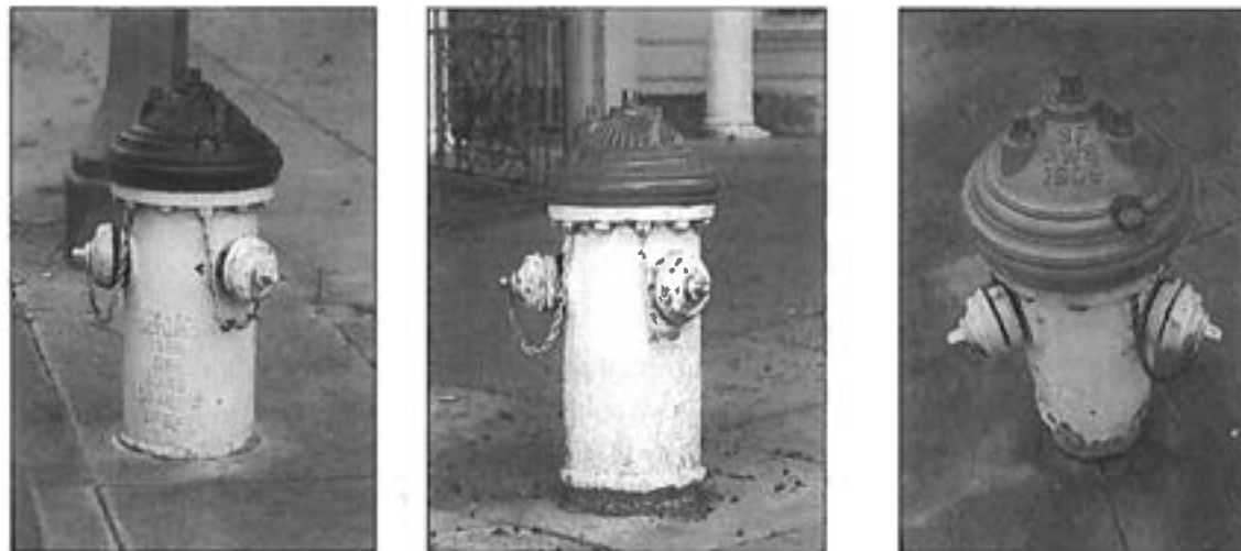
Figure 10 Color-coded SF AWSS hydrants
