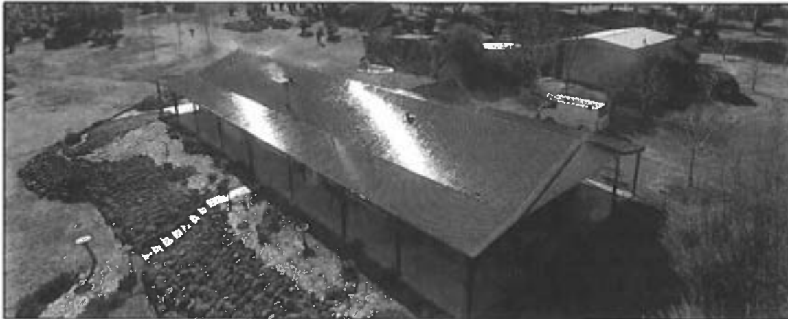
Figure 16 Rooftop Sprinklers on Residential Building
