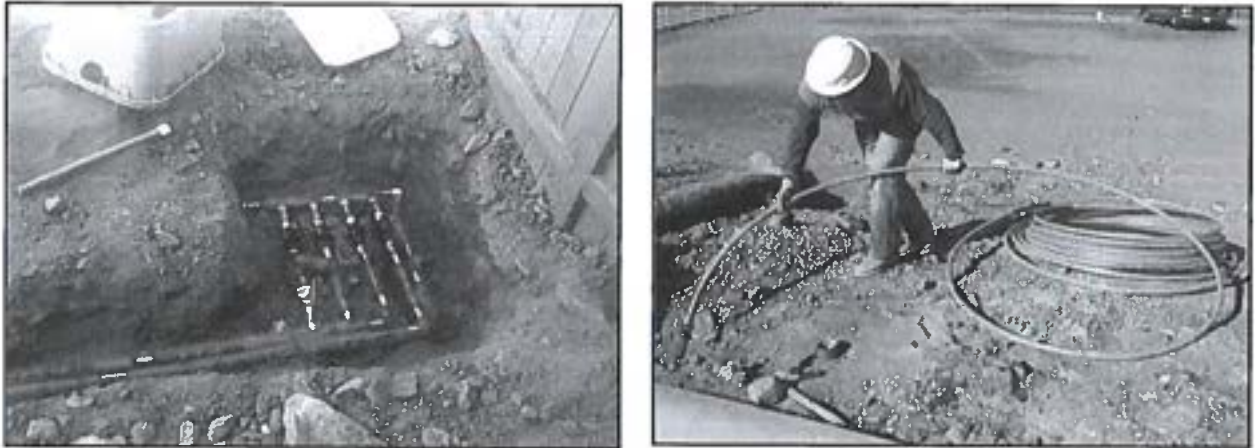
Figure 5 Recycled Water Residential Irrigation Installation, El Dorado Hills, CA
