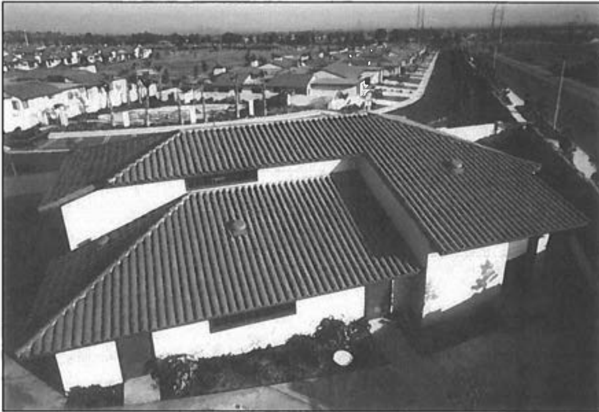
Figure 2 Satellite Water Reclamation Plant, San Bernardino County, CA, image circa 1981
