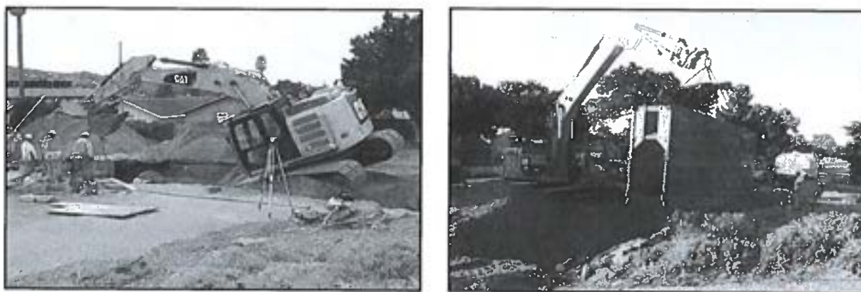
Figure 1 Gravity Collection Construction, San Luis Obispo County, CA
