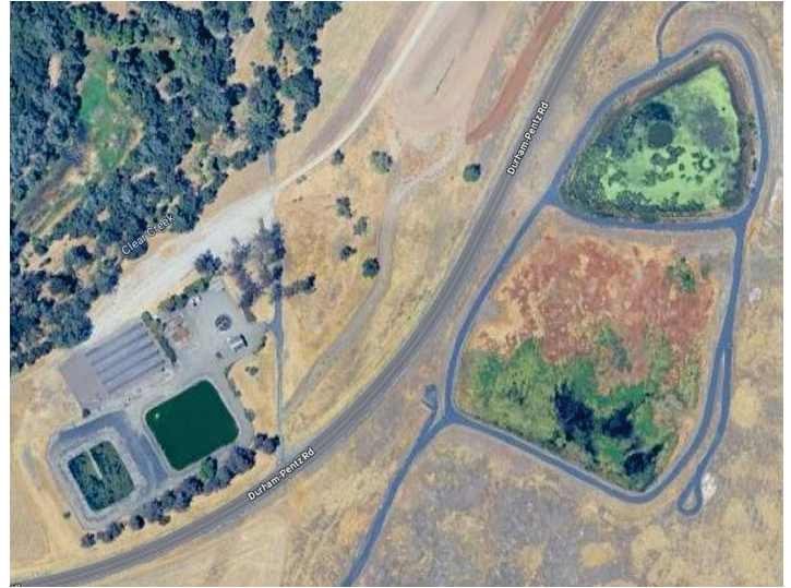
Treatment plant (left) and discharge ponds (right)
