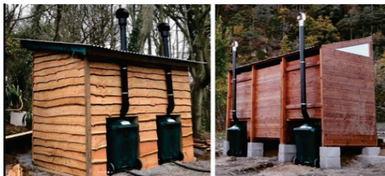
Composting toilet installation
