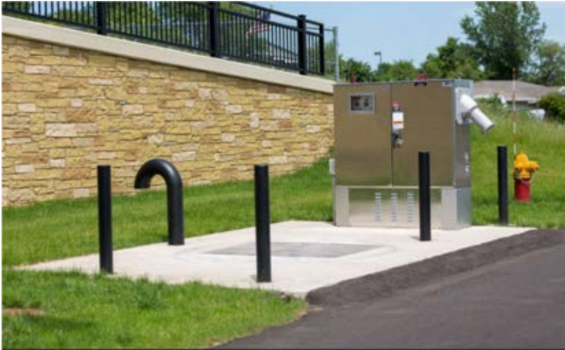
Figure 2-9. Example Transition Chamber with Vehicular Bollard Protection
