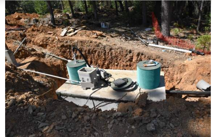
Septic Tank & STEP pipe
