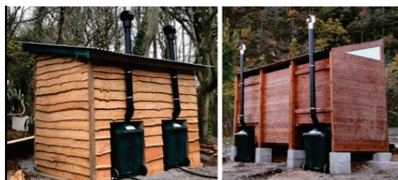
Composting toilet installation
