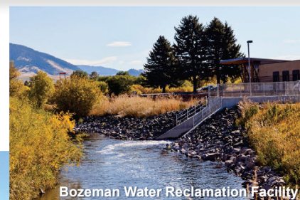
Bozeman Water Reclamation Facility
