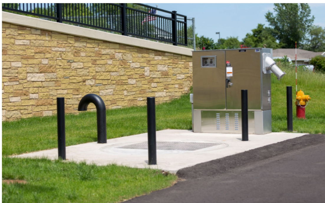
Figure 2-9. Example Transition Chamber with Vehicular Bollard Protection
